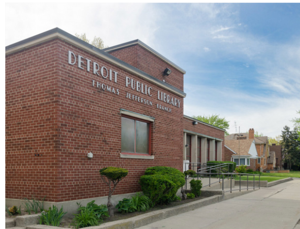
Jefferson Branch Library. Image courtesy of Detroit Public Library
