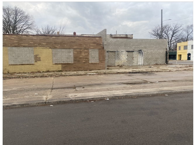
The partially-demolished building at East Warren Avenue and Bedford. Image courtesy of Jeffrey D. Lewis II
