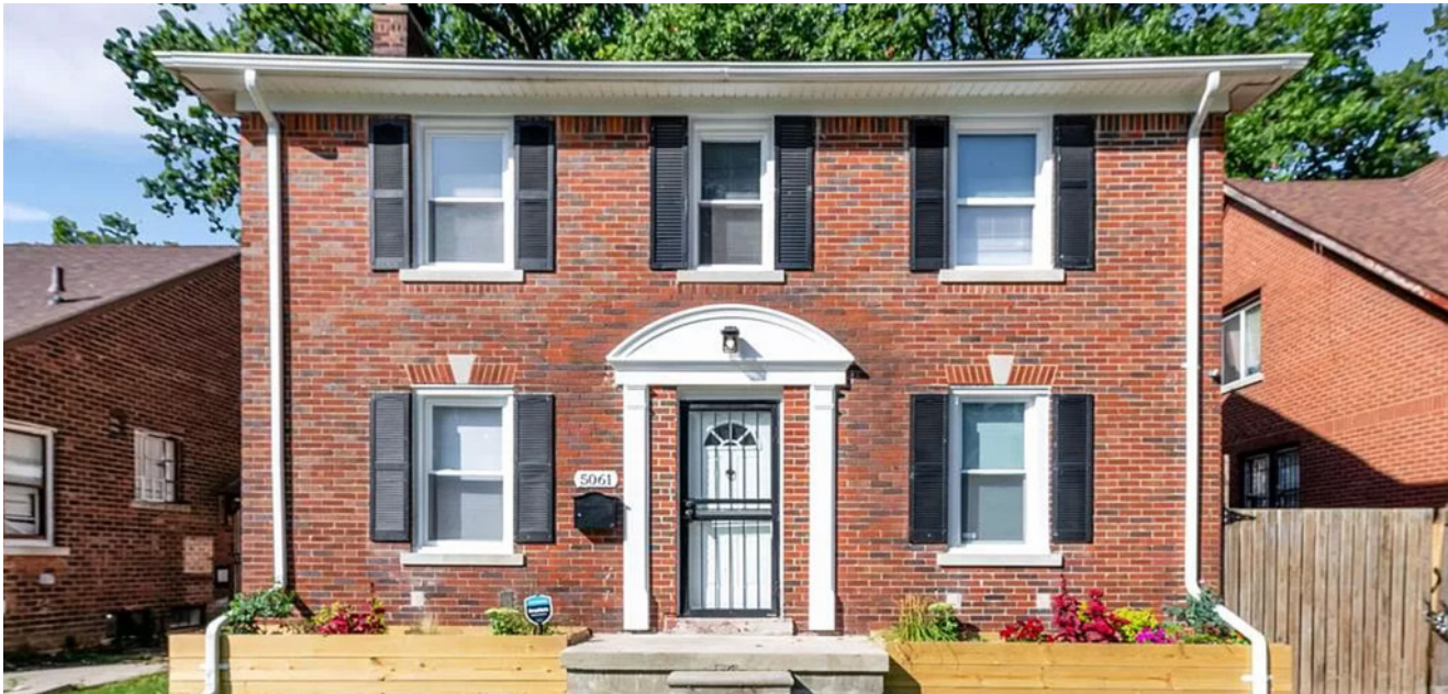
U- SNAP BAC will look to renovate a previously owned DLBA home similar to this one in Morningside. Image courtesy of Zillow
