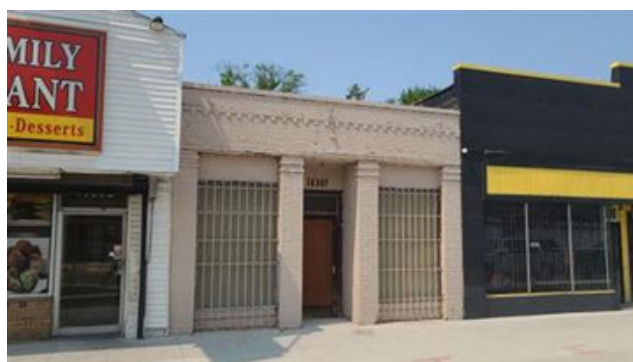
An after photo of 16357 E. Warren Avenue freshly painted. Image courtesy of Susan Newell
