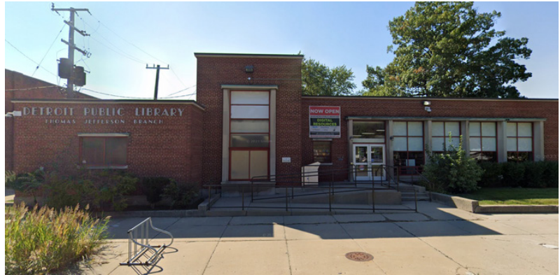
Jefferson Branch Library. Image courtesy of Google Street View
