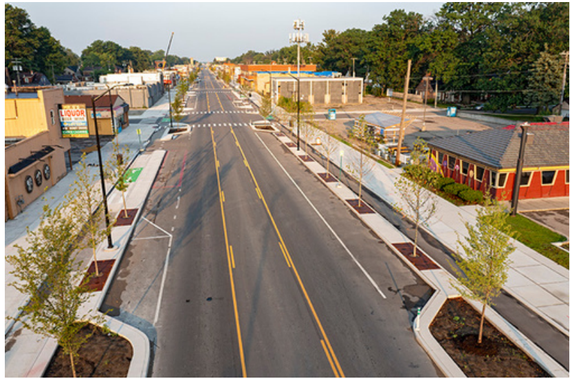
An aerial shot of the streetscape improvements to East Warren Avenue. Image courtesy of Jim West
