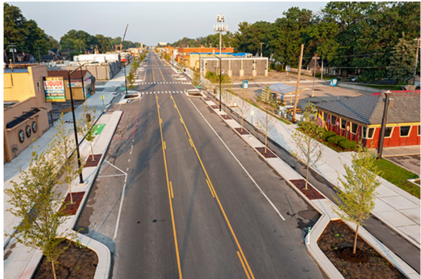
An aerial shot of the streetscape improvements to East Warren Avenue. Image courtesy of Jim West
