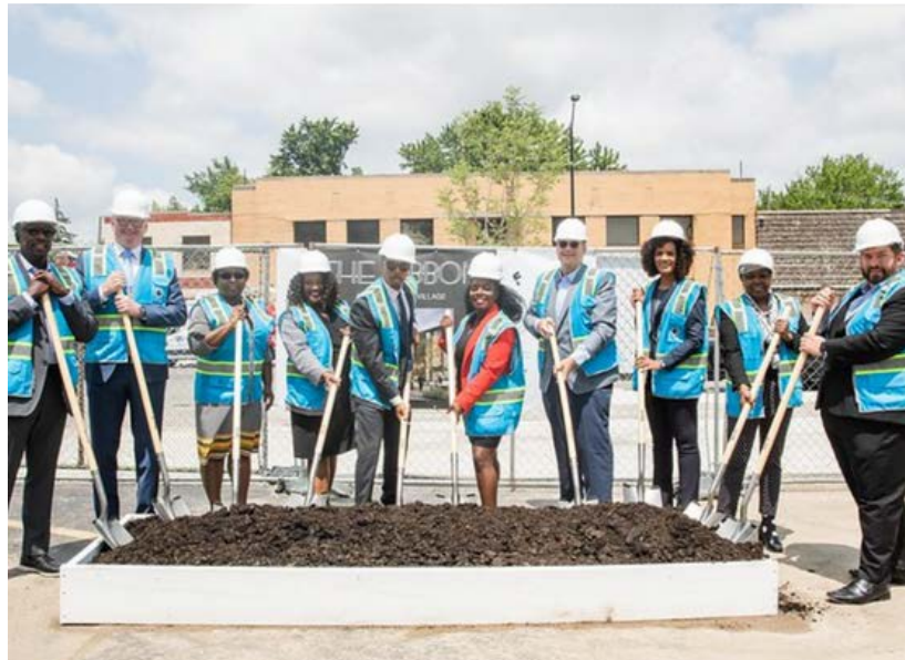
Officials celebrate the groundbreaking of The Ribbon. Image courtesy of the city of Detroit
