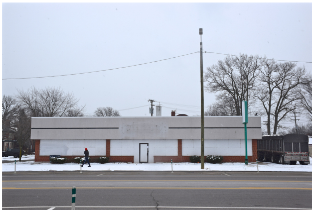
The former Charter One bank will be redeveloped into The Ribbon. Image courtesy of Edward Carrington
