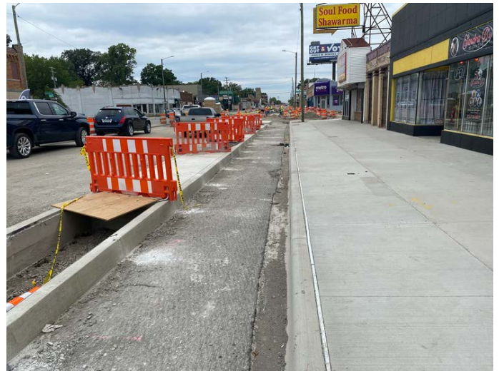
With the addition of the raised platforms, bicyclists will be protected from other methods of transportation. Image courtesy of Jeffrey D. Lewis II
