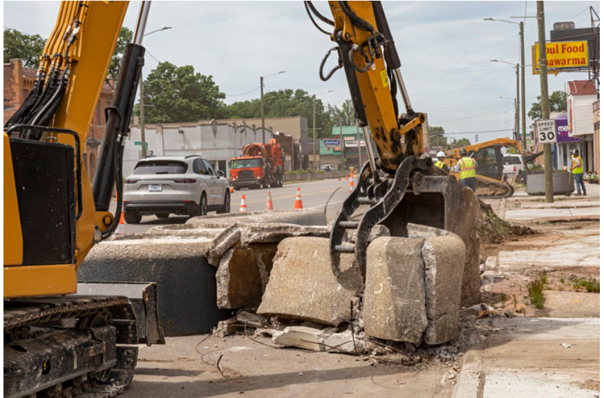
Excavators dismantling the planters. Image courtesy of Jim West
