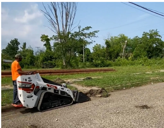
The removal of sod along the curbside on Cornwall St. Image courtesy of Charon and Gaston Nogues
