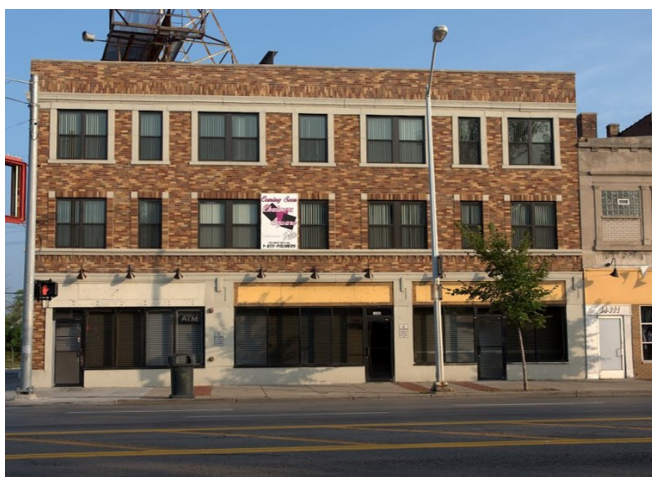
Renovated, two-story mixed-use on East Jefferson Avenue. Image courtesy of the EWCP
