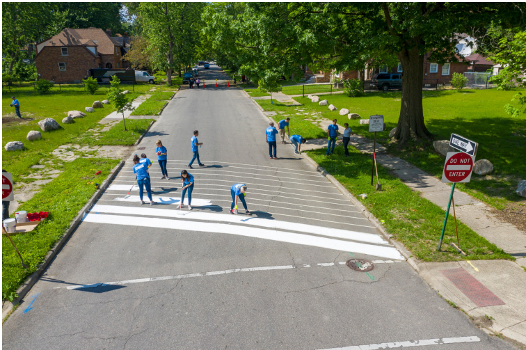
SAY Detroit volunteers installing streetscape art. Photo by Jim West.
